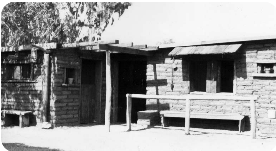
Outbuildings at the Wieghorst home circa 1950. The stable and cantina, including much of the original adobe walls, will be restored and re-assembled next to the museum building on Rea Avenue.
